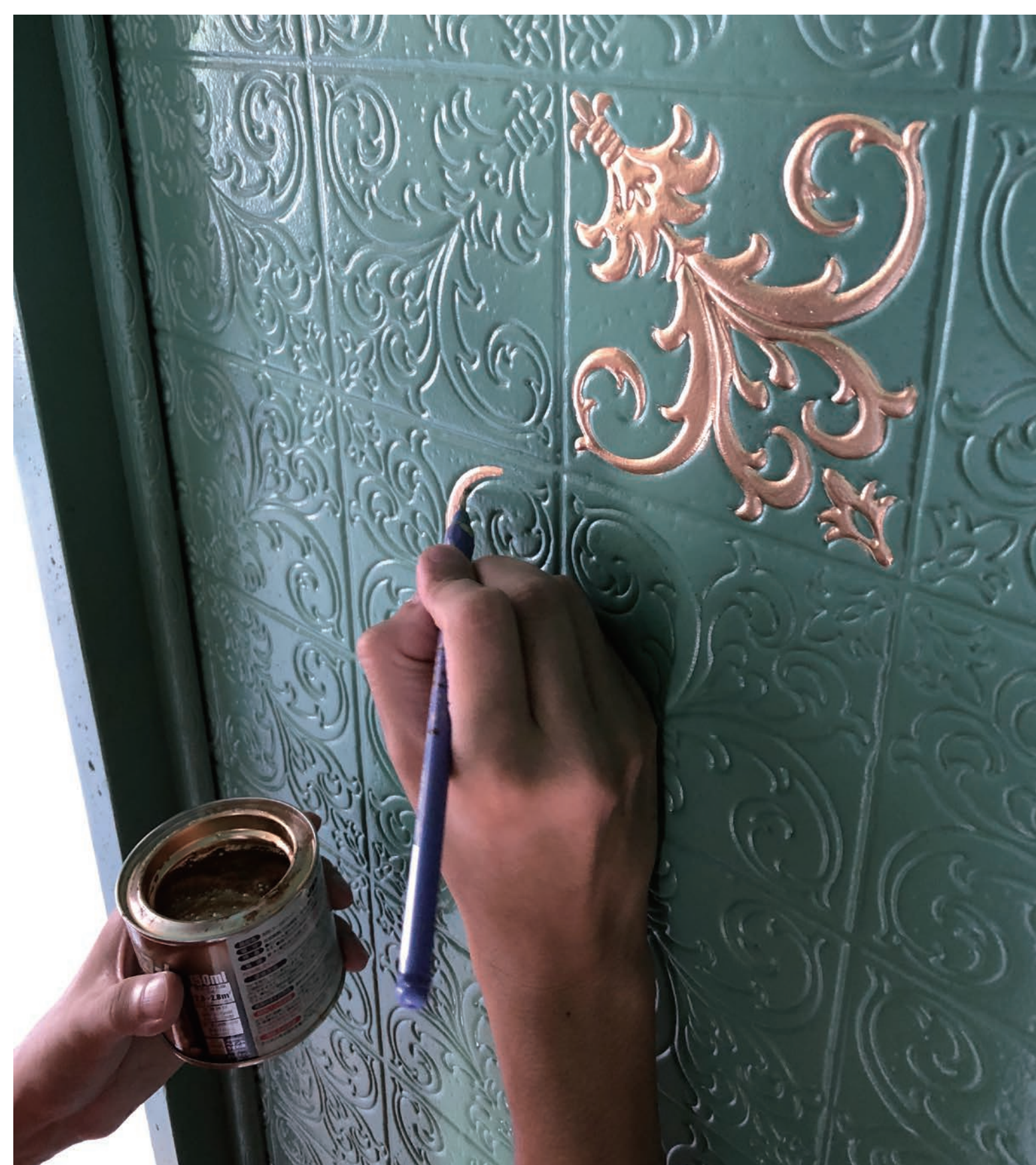
Painting existing off-the-shelf wallpaper. An irrational method in the concept of new construction may be rational in the renovation.
