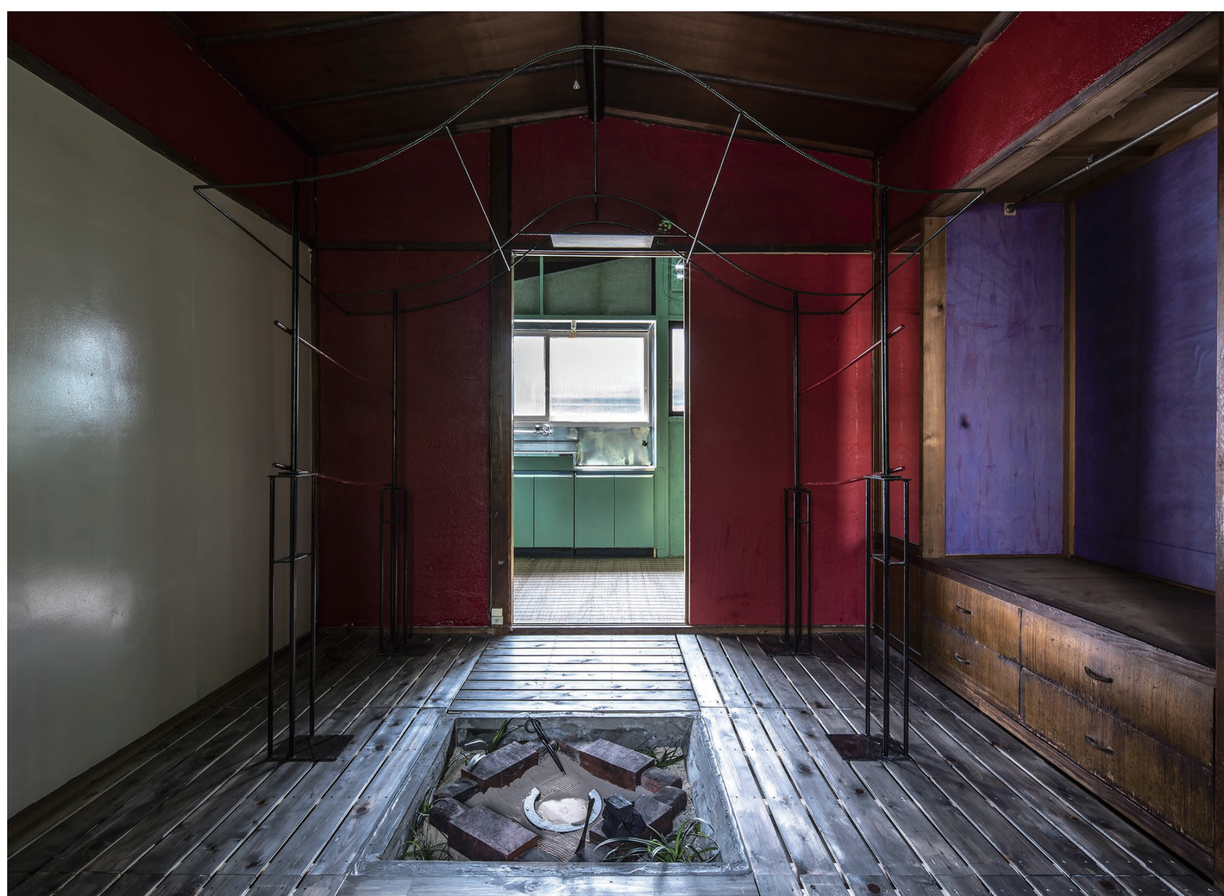
Japanese-style room. The existing tatami mats have been peeled off and replaced with floors made from ready-made drainboards. Taking advantage of the low size of the closet before the war, it was diverted to the alcove. (photo© Takuya Seki)
